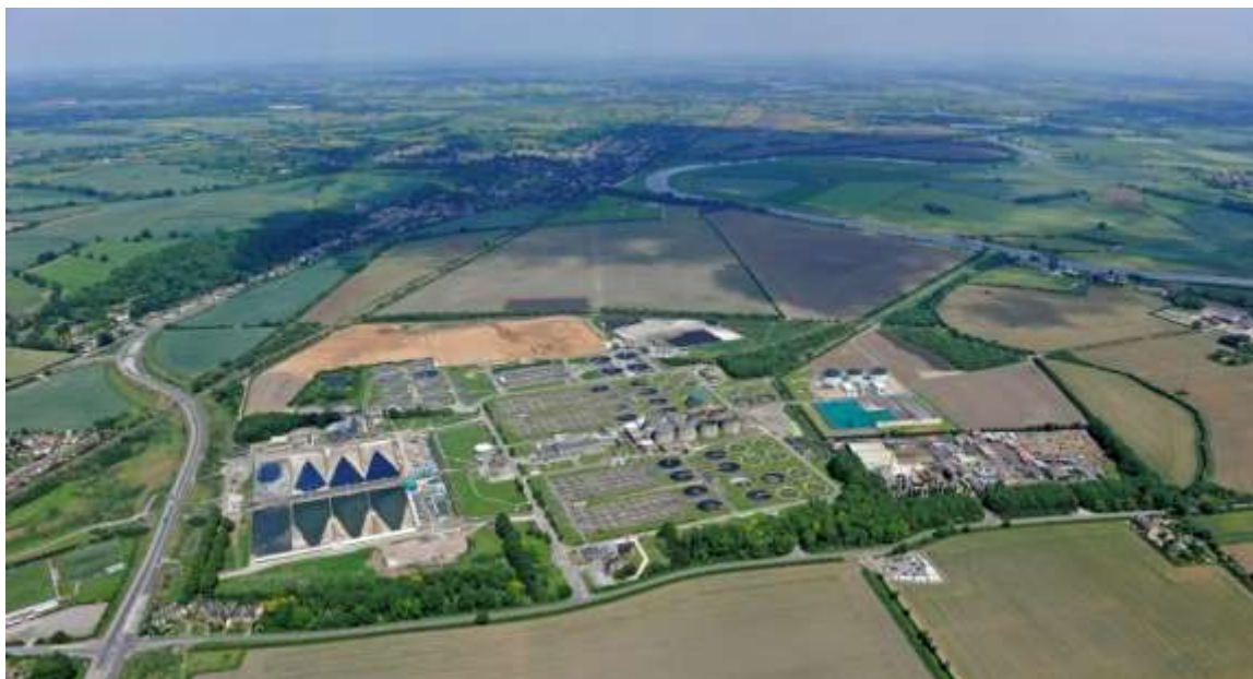
Figure 1: Stoke Bardolph STW pictured before capital works
