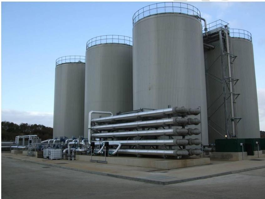
Figure 3 Enhanced enzymic hydrolysis reactors at the Great Billings sludge treatment centre operated by Anglian Water and achieving a 6-log removal of *E. coli*
